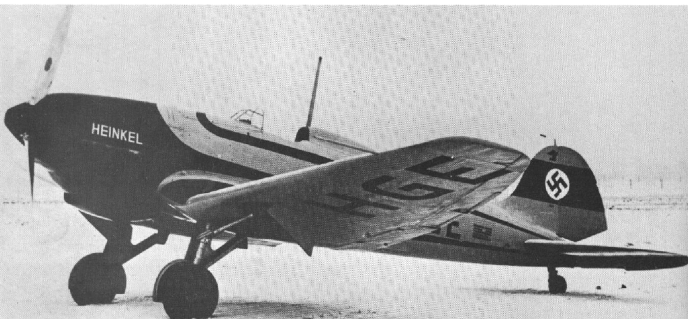
The airframes of the HE 112 V-1 and V-2 were almost identical. Installation of the German Jumo 210 did, however, change the exterior shape.
