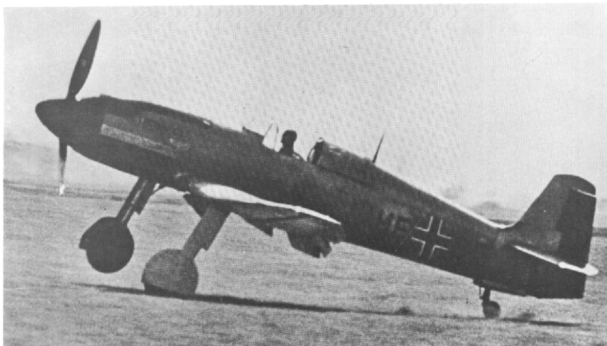
He 100 V-3. Note short wing and sharp curved two-piece windshield.
